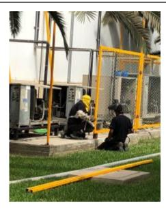
Observed during the site tour, two maintenance workers in the labour of welding that do not have the right PPE (mask for gases).
